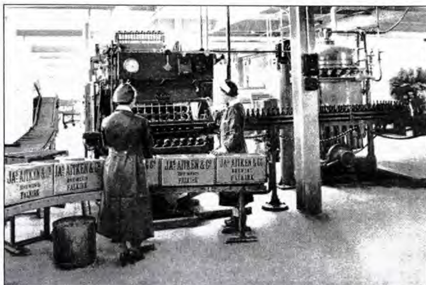
Aitken's bottling hall in 1940 (By courtesy of Falkirk Council Museum Services)
